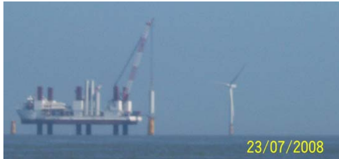
Windfarm under construction off Skegness.
